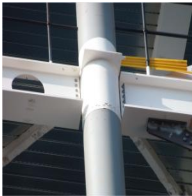
Fig 9: Typical Beam-Column Shear Connection Detail
